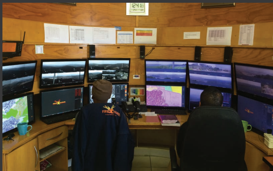
The camera detection control room
