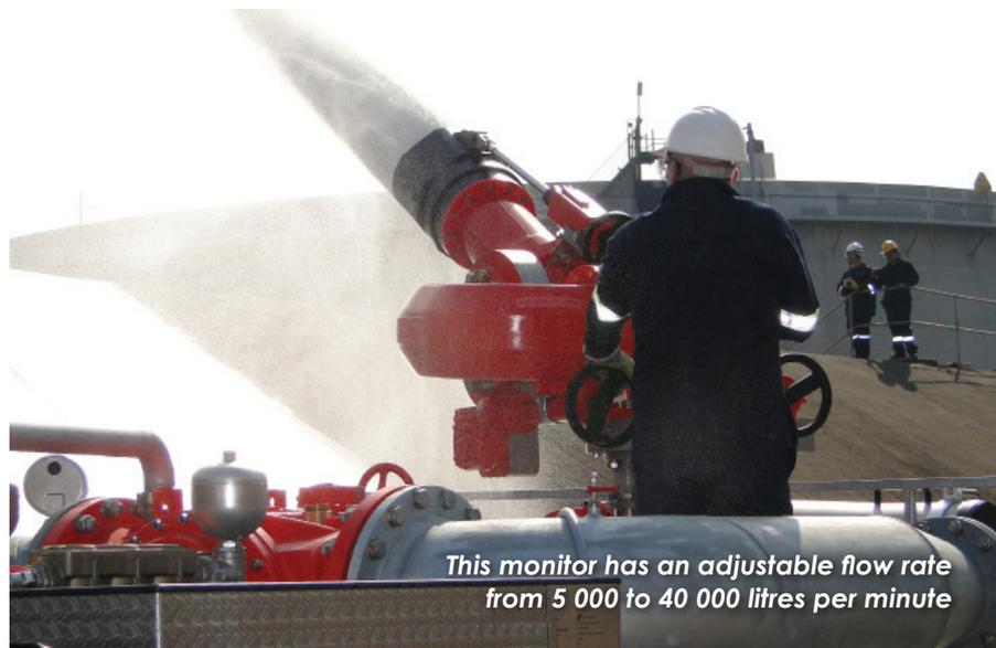
*This monitor has an adjustable flow rate from 5 000 to 40 000 litres per minute*
