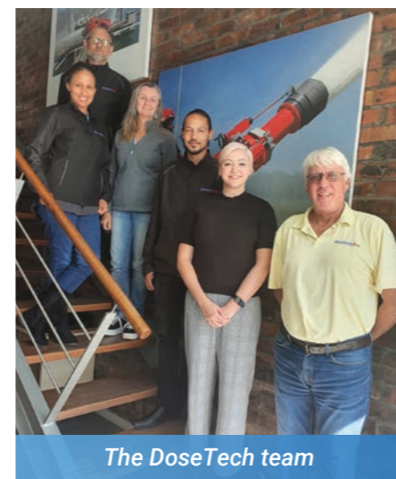
Commissioning Cape Town harbour sea water FD20000/1/3 foam proportioner with Ingo Wosch and Heinrich David, the founder of FireDos (on the left), Mike Feldon, JB Potgieter and Greg Buchanan from DoseTech
