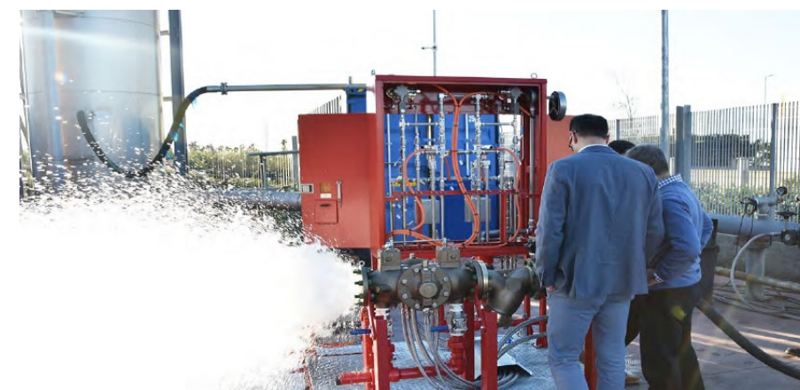
The VDD has been designed to comply with the requirement of S001 granting continuous operability even during maintenance
