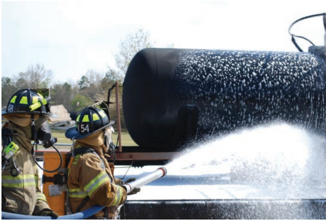
Dealing with a fire impingement on an LPG vessel will require immediate and massive cooling of the entire surface
