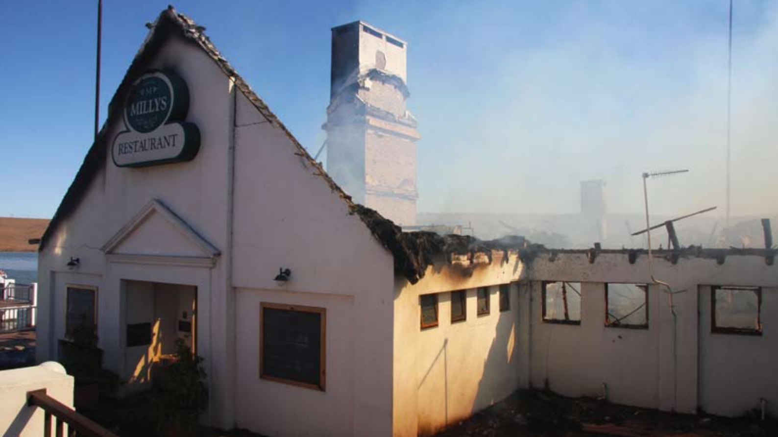
Photographs courtesy of Highlands Herald
