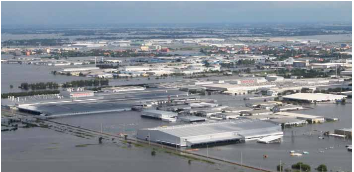
Flooding of Rojana Industrial Park, Ayutthaya, Thailand
