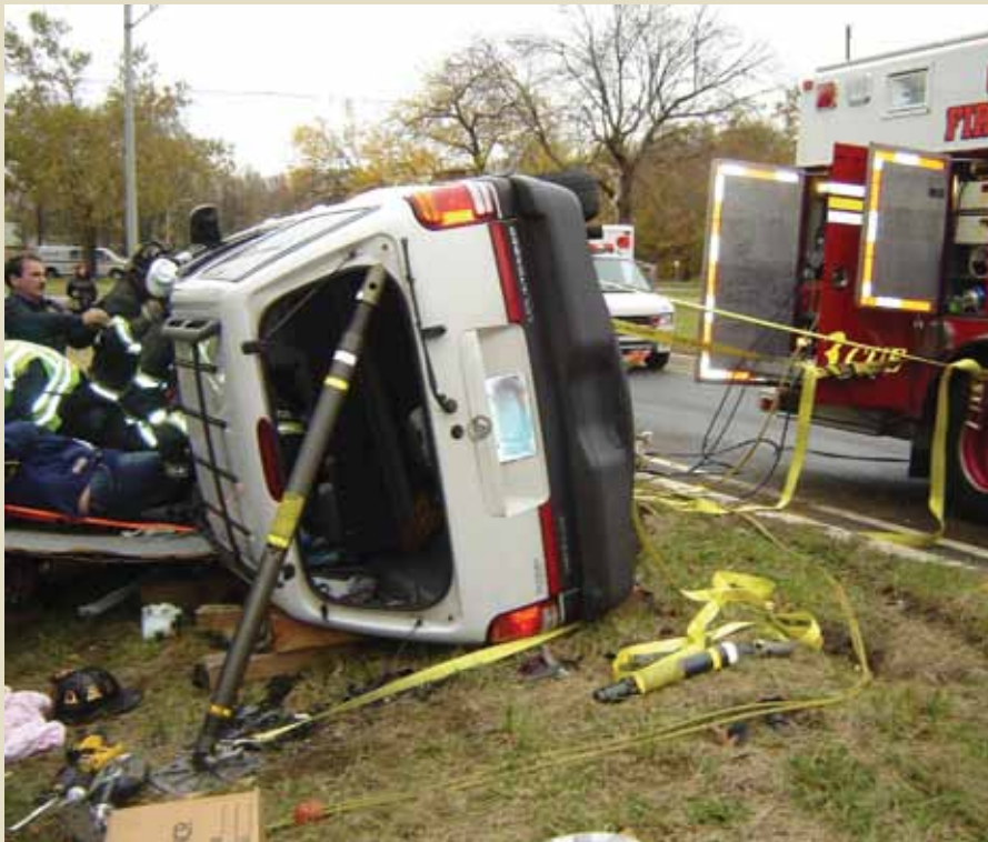
Hydraulic rescue tools used to extricate the patients through the roof of the vehicle
