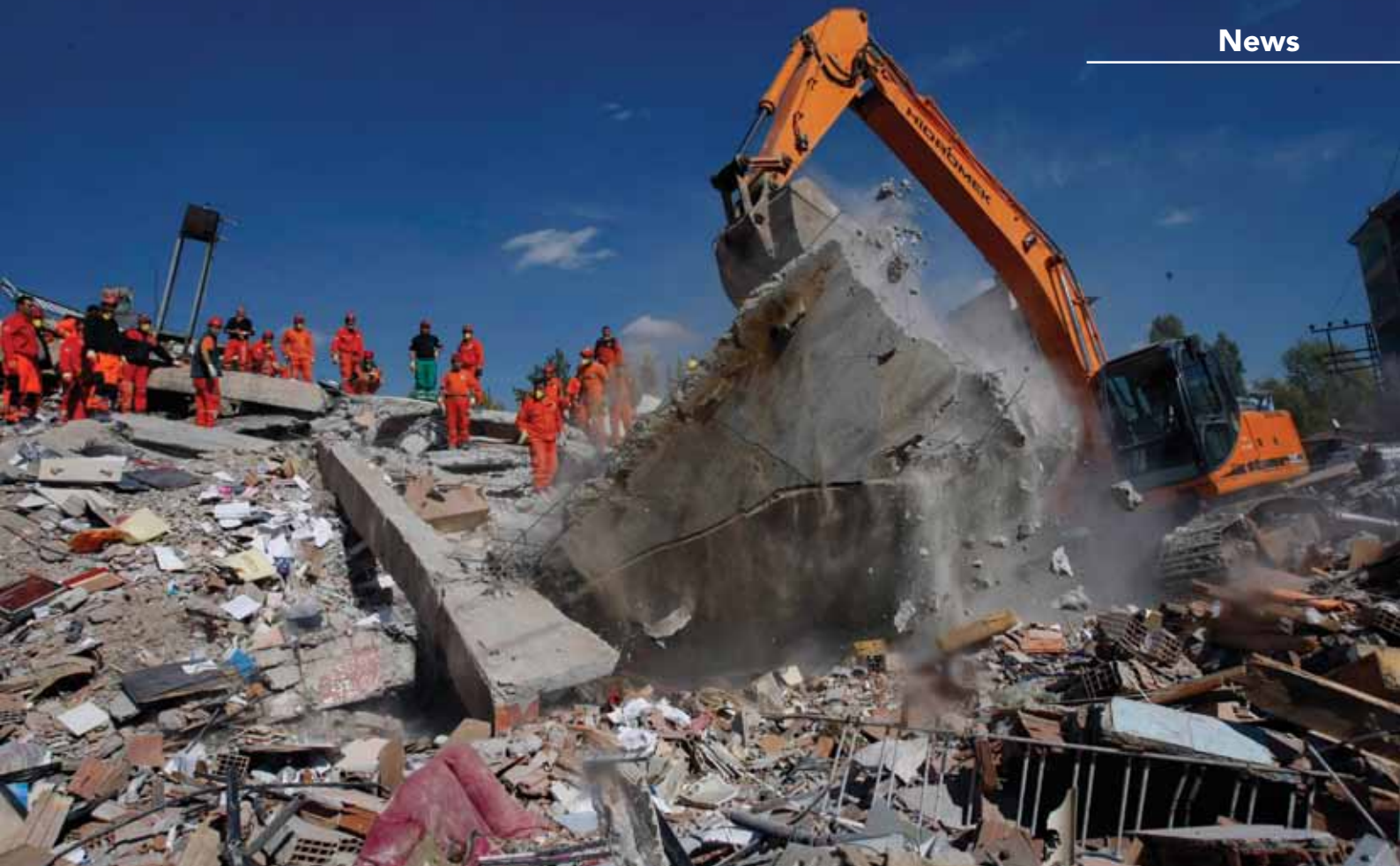
Earthmoving equipment assisted in the rescue operations
