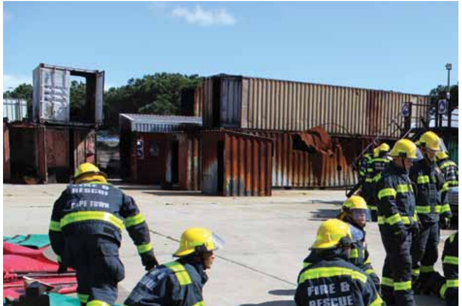
The modernised Epping Training Academy
