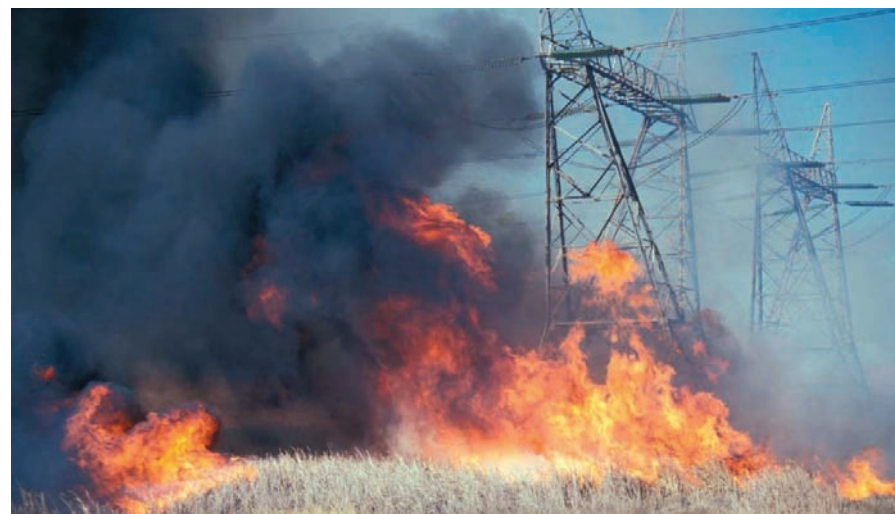
Figure 1. Grass fires burning underneath Eskom power lines
