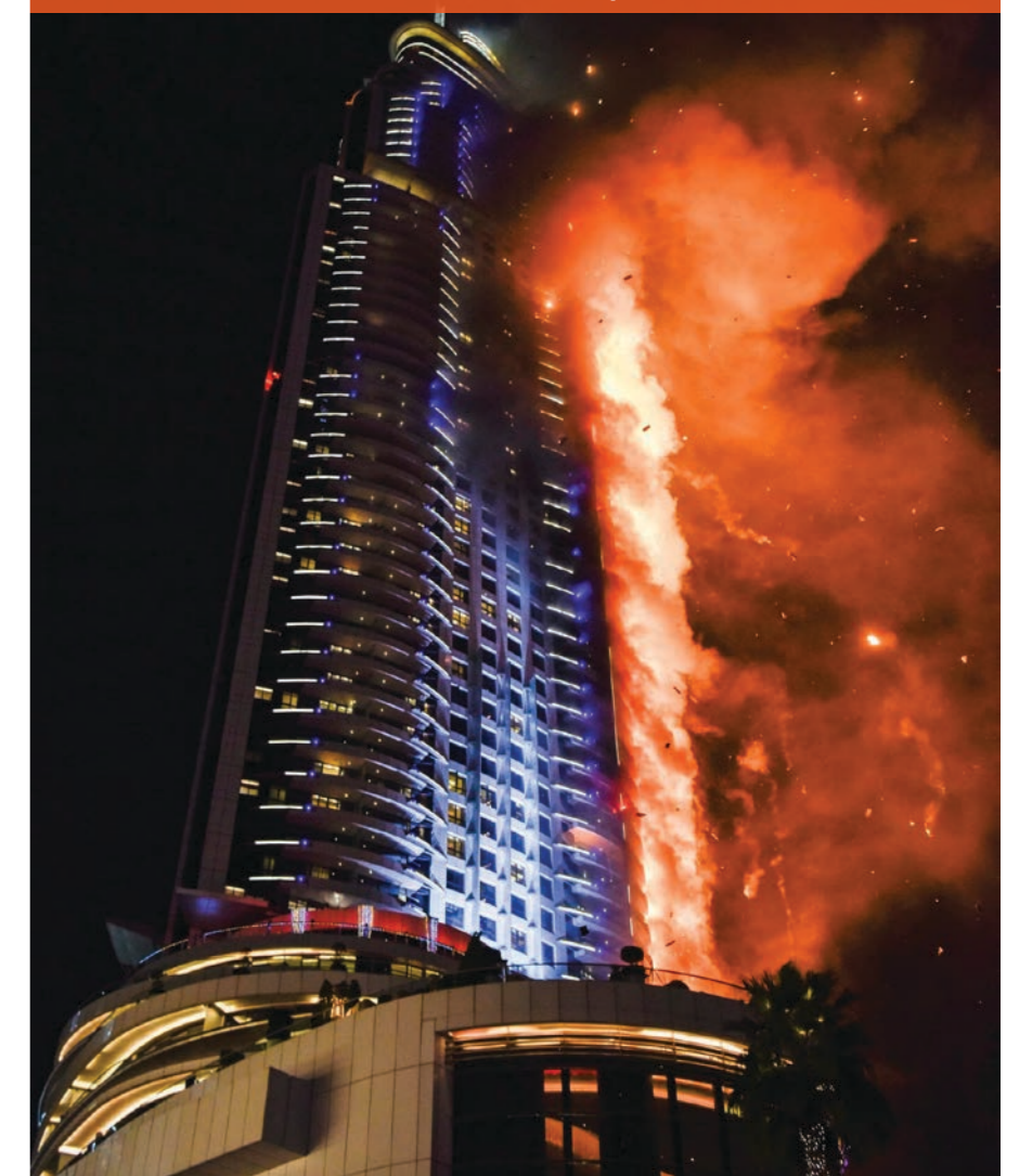
High-rise fires present unique challenges due to the height of the building, the potential for rapid fire spread and the need for effective evacuation and rescue operations
