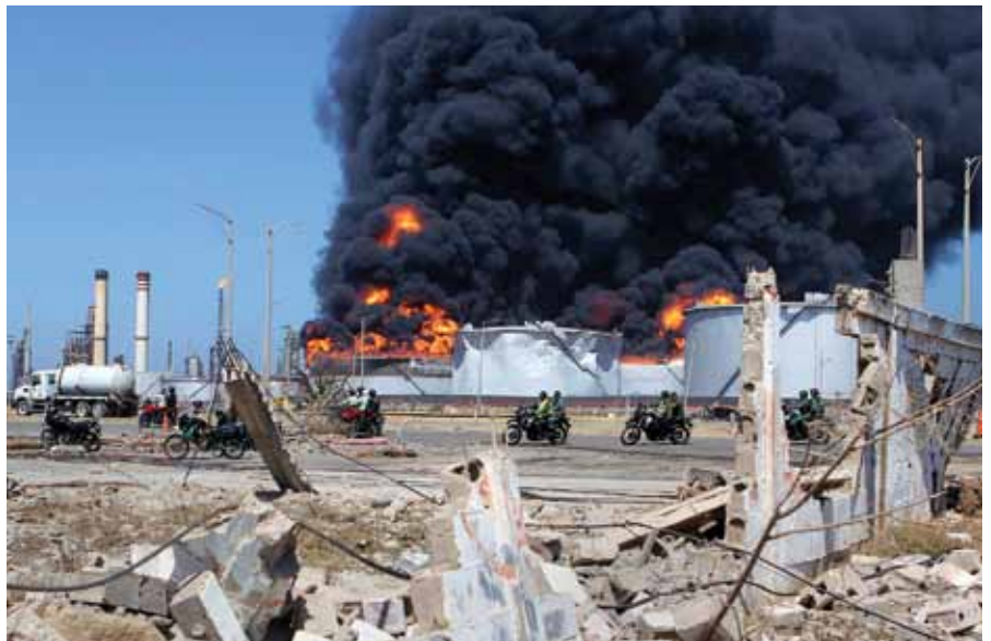
Fuel storage tanks on fire, a day after an explosion
